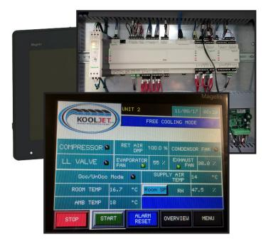
KoolJet provides a comprehensive yet user-friendly interface to the control system settings. The "Master" and all "slave" units are accessible from one screen that is connected using common control wires. Each KoolJet slave can have its own temperature and humidity settings. This strategy maximizes the ability to store some produce for short term and some for long term.
