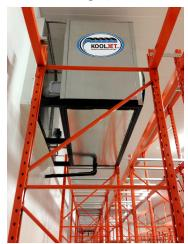
Indoor units are designed to move massive amounts of cold air in order to rapidly freeze commodities.
