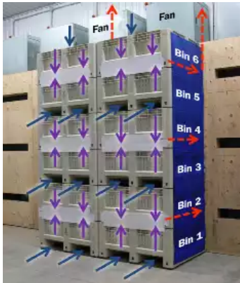
Figure 4. This serpentine horizontal/vertical airflow system has centrifugal fans inside metal housings above a plywood plenum. These fans pull refrigerated air through "hot" tree fruit in plastic bins. Each stack of six bins is independent. Three forklift openings across from wall slots are closed off with coverings. This compels cold air to enter through the remaining three open forklift openings and travel up or down through the fruit via slots in the bin floor. As the air warms (purple arrows), it is directed back into the storage room (red arrows) towards the evaporator coils to be re-cooled. Bins are tightly stacked so no air can short-circuit through the bins' side vents. If stacks are missing, a tarp is installed to prevent short-circuiting. This tarp can be seen covering the sides of the right column of bins. The system shown here is under construction, as foam padding around the slots is to be installed. (Photo by Hugh Fraser, OMAFRA)
