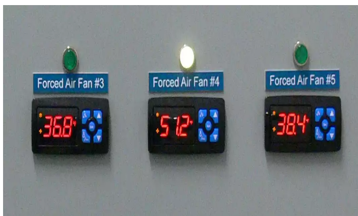
Figure 6. Sensors monitor "warm" air temperatures (°F) exiting the column of bins in the serpentine horizontal/vertical airflow system in Figure 4. At the time of this picture, cold air entering Forced Air Fan #4 was 35.6°F (2°C) and the internal temperatures of three individual, equally sized pears being monitored were 59°F (15°C), 67°F (19°C) and 68°F (20°C) along the cooling path, averaging 64.4°F (18°C). Fruit started at about 71.6°F (22°C), so the temperature at Fan #4 (51.2°F; 10.7°C) is about halfway between the cold air entering at 35.6°F (2°C) and the average internal temperature of cooling fruit at 64.4°F
